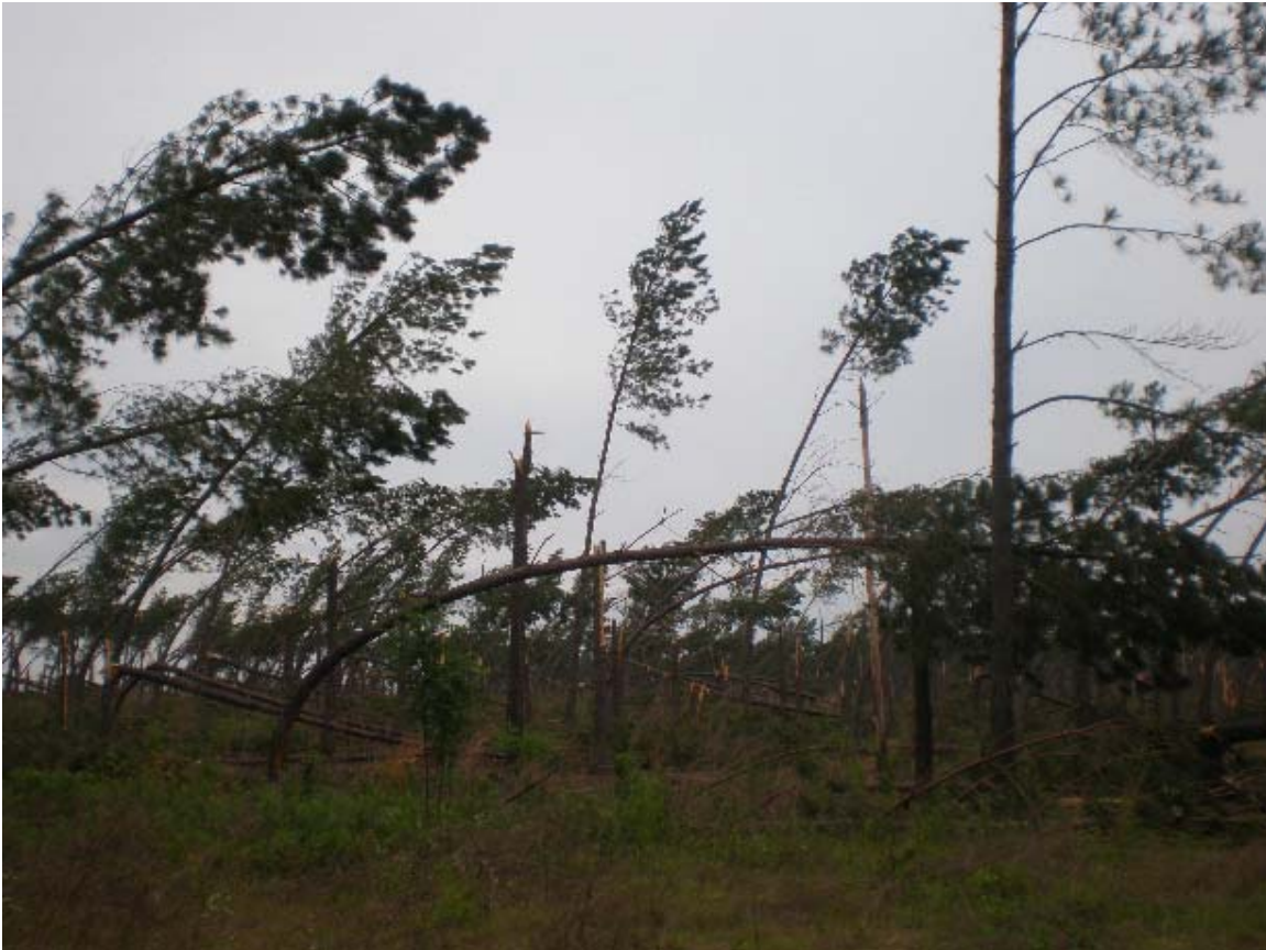
Photo 3. Severe damage pine stand; less than 30 trees per acre standing in good condition
