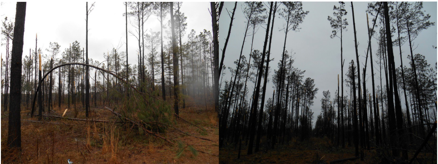
Photo 1 and 2. Examples of a severely damaged pine stand (left photo) with less than 100 good crop trees per acre and a moderate to severely damaged pine stand (right photo) with a marginal number of crop trees left per acre.
