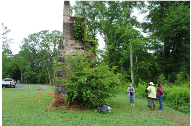
Bridge Pier "before" 2018 project
