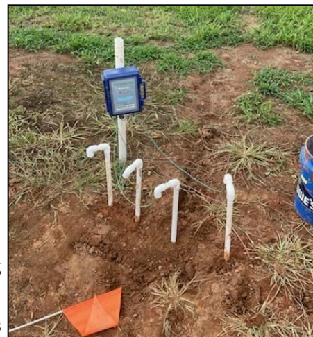
Figure 4. Moisture sensors placed Crowe family orchard in Oconee County, GA.
