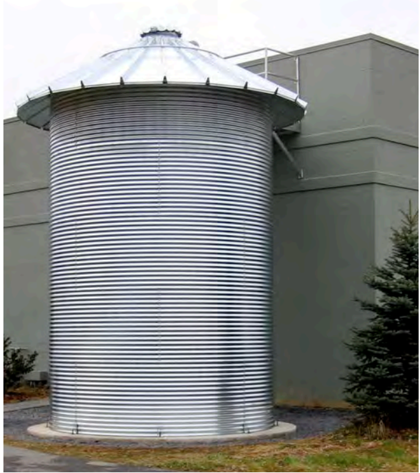
Figure 4-14 Corrugated steel tank
