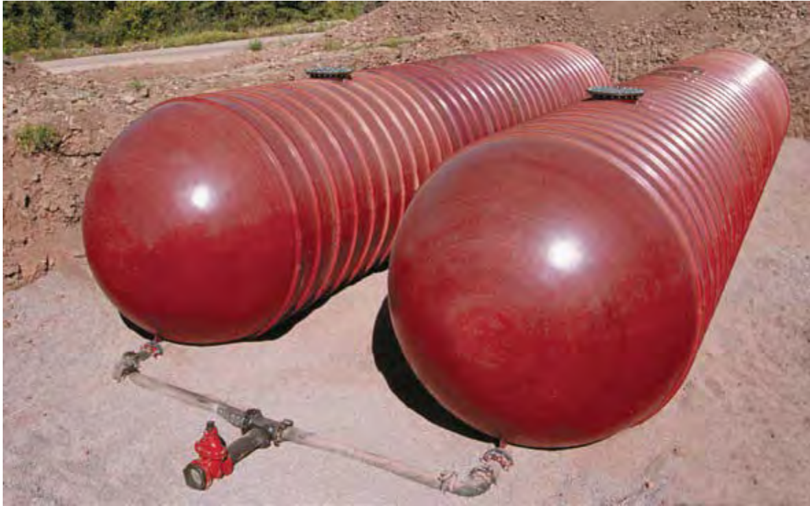
Figure 4.12 Below ground fiberglass tanks
