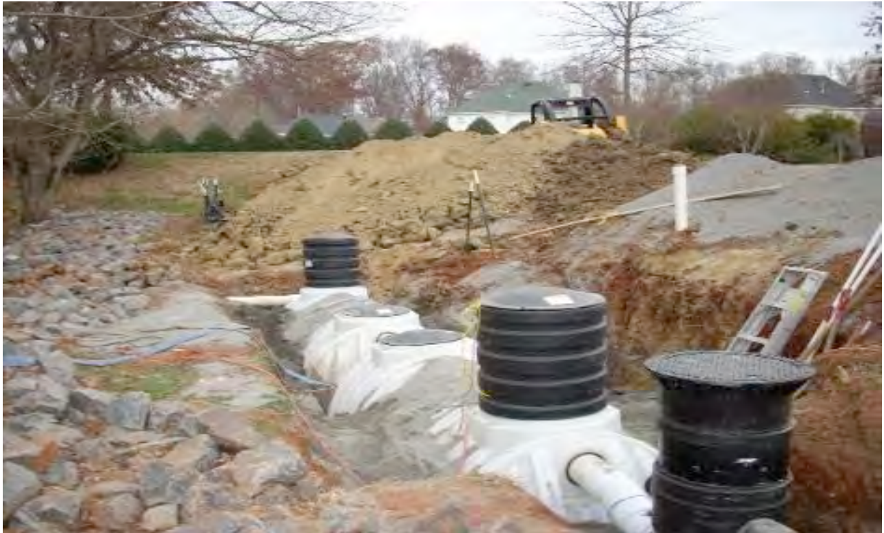
Figure 4.13 Below ground polypropylene tanks
